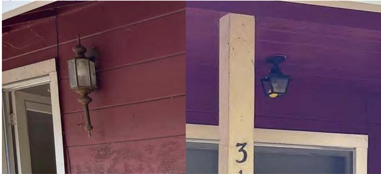
EXISTING SIDE EXTERIOR LIGHTING
